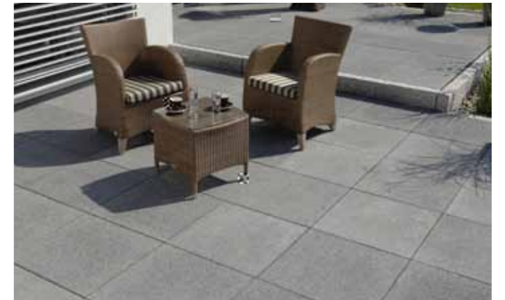
Shot blasted slabs
